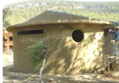
(Left) Construction of a public shower on the beach.
